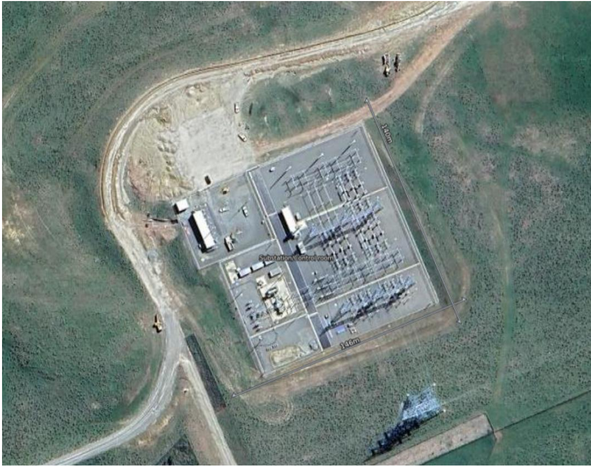
Figure 15: Managed area around the Control Room and substation
