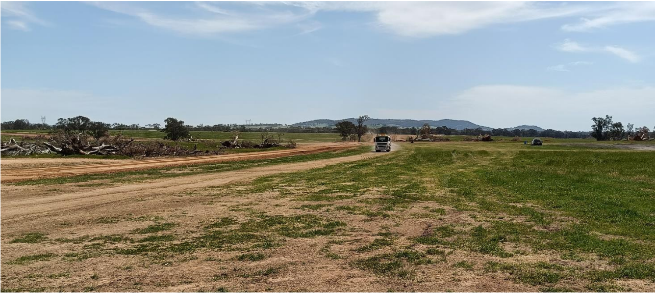
Photograph 3.6 Water Cart in operation on active road construction area
