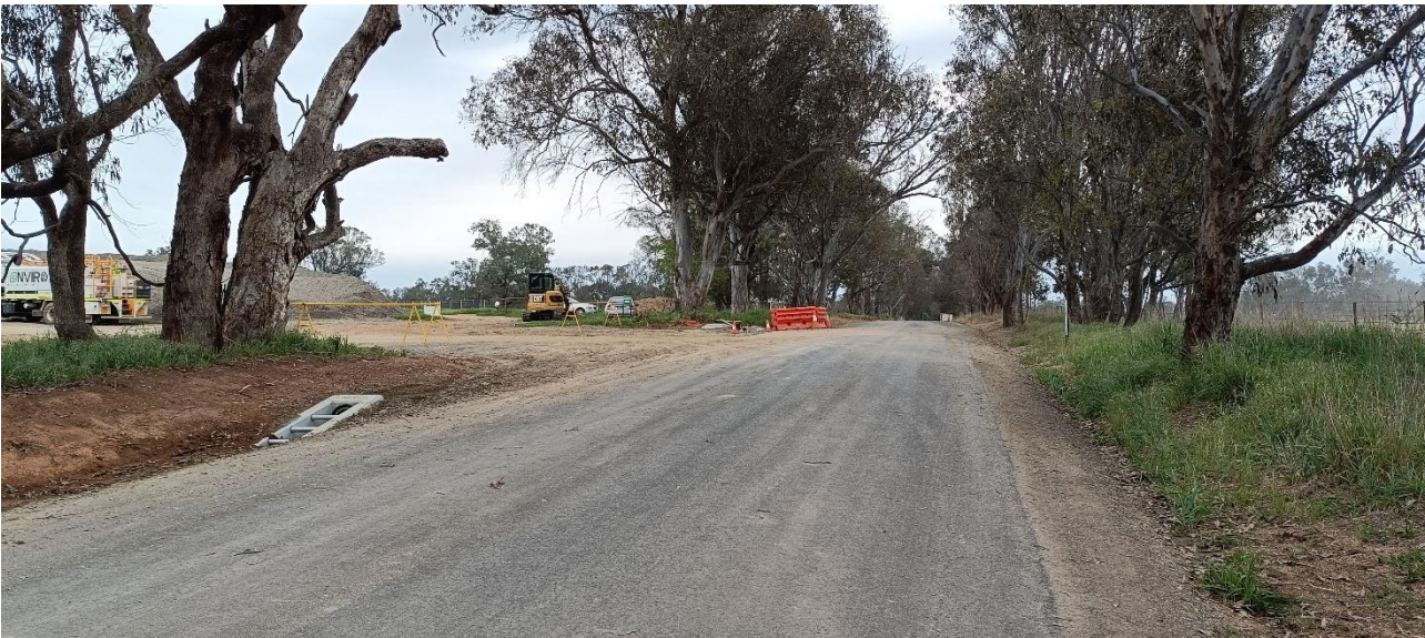
Photograph 3.5 Ortlipp Road access point
