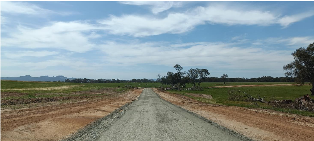
Photograph C.2 Typical road under construction
