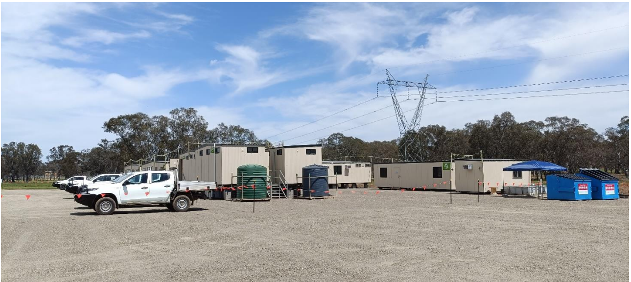
Photograph C.3 Site office and laydown area setup
