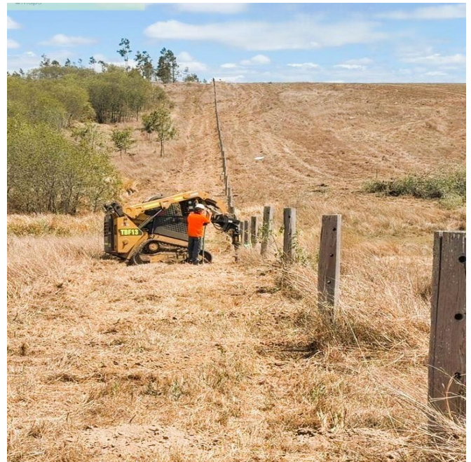
Figure 1: Post holes being prepared ahead of security fencing installation along the project's Southern boundary
