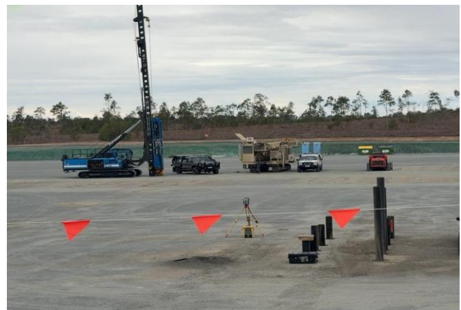
Figure 3: Pile driving has begun at the BESS pad. The piles once in place support the modular batteries to be stood on the pad
