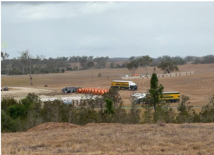
Figure 2: Laydown area adjacent to Gigoomgan Road for construction material delivery
